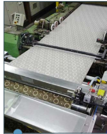
Stenter frame installation
